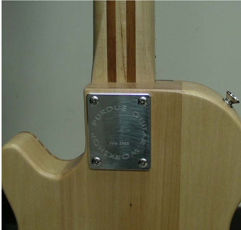
Figure 43 – Neck Fixed to Body with a Neck Plate and Screws
